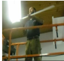
B. J. Williams prepares to install a light tube.
